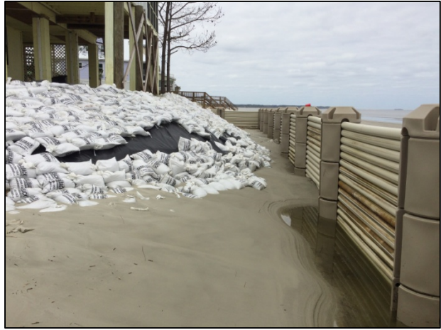
Figure 3: Harbor Island WDS location after WDS installation (left) and after new sandbags (right).
