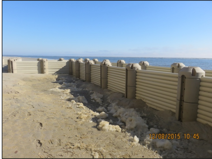
Figure 13: Small mounds of sand that have been able to move landward through the Ocean Club WDS in December 2015.
