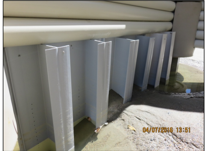
Figure 17: The actual Vertical Porous Panels that were installed at the Ocean Club WDS (left). Note that very small drill holes were used instead of slots, resulting in a VPP with minimal porosity (right).
