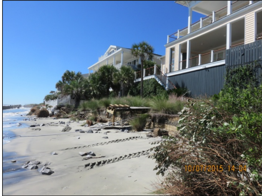
Figure 2: Scarp erosion landward of the Beachwood East WDS during storm conditions before the placement of emergency sandbags. This was approximately 1 month after the WDS was installed.
