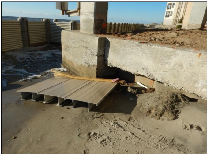
Figure 18: A Vertical Porous Panel that was dislodged by waves at the Ocean Club WDS in February 2016. Photo was taken by Stantec.
