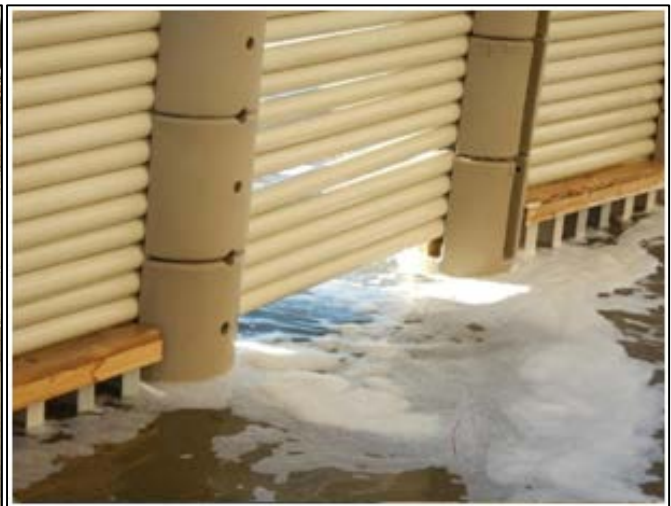
Figure 18: A Vertical Porous Panel that was dislodged by waves at the Ocean Club WDS in February 2016. Photo was taken by Stantec.
