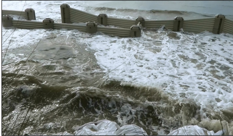
Figure 7: Waves re-forming and breaking on the landward side of the Beachwood East WDS. Video screen-grab from September 29, 2015.
