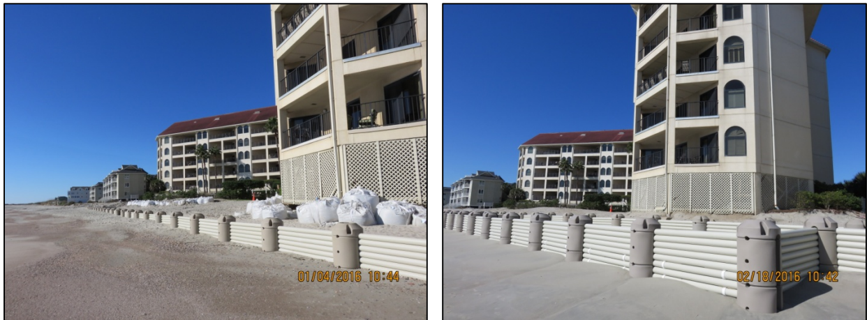
Figure 6: Seascape Villas WDS location before 2 nd tier installed (left) and after 2 nd tier installed (right).
