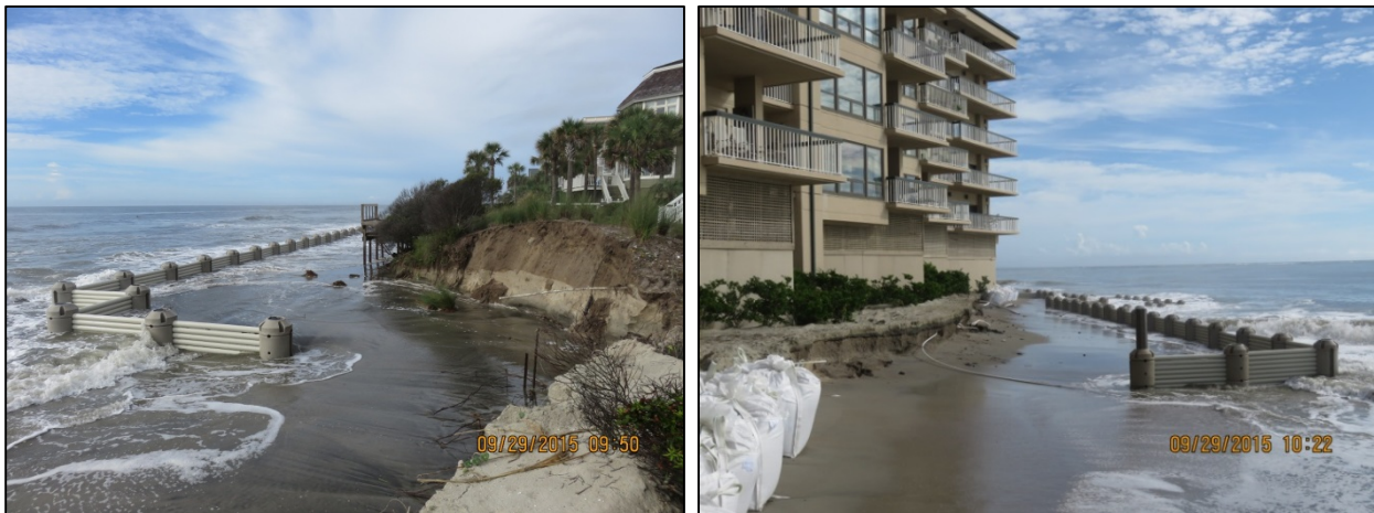
Figure 22: Erosion at the northeastern end of the Beachwood East WDS (left) and the southwestern end of the Ocean Club WDS (right).
