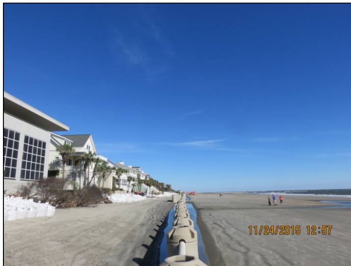
Figure 14: Scour (trenching) on the seaward and landward sides of the Beachwood East WDS.
