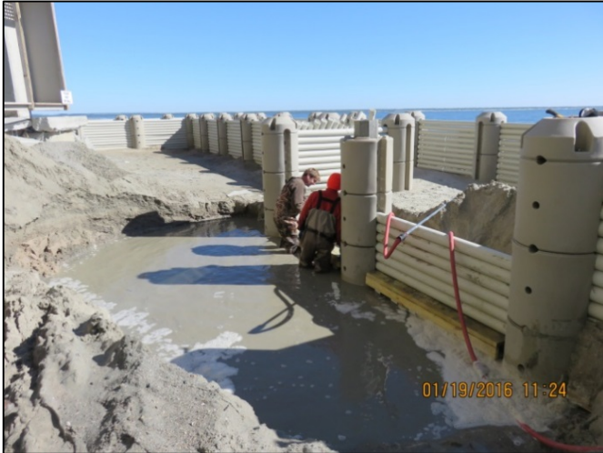
Figure 17: The actual Vertical Porous Panels that were installed at the Ocean Club WDS (left). Note that very small drill holes were used instead of slots, resulting in a VPP with minimal porosity (right).
