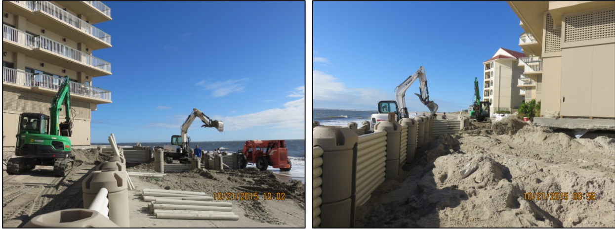
Figure 21: Adjustments to the Ocean Club WDS being made by The Citadel research team after Hurricane Joaquin in October 2015.
